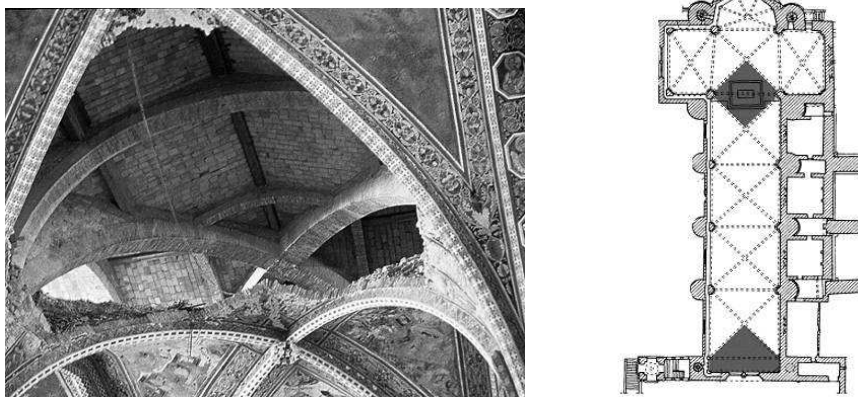
Fig. 1 – St. Francesco d'Assisi basilica. Damages on the vault after the 1997 earthquake.
