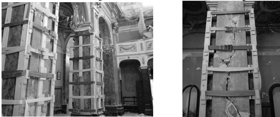
Fig. 7 – Observed damages after the 2009 seismic event on rubble masonry pillars of St. Gemma church (SGM) in Goriano Sicoli (AQ).
