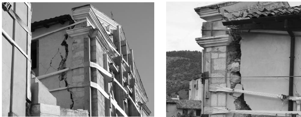
Fig. 8 – Façade overturning in St. Gemma church (SGM) in Goriano Sicoli (AQ)
